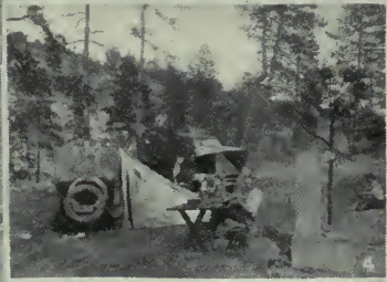
1 On the Montana Route of National Parks Road 2 Overland Park, Denver, Colorado 3 Southern California Public Camp Ground 4 Public Camping Park, Spokane, Washington
